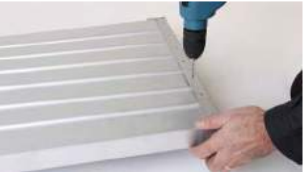
2. Drill rivet holes
